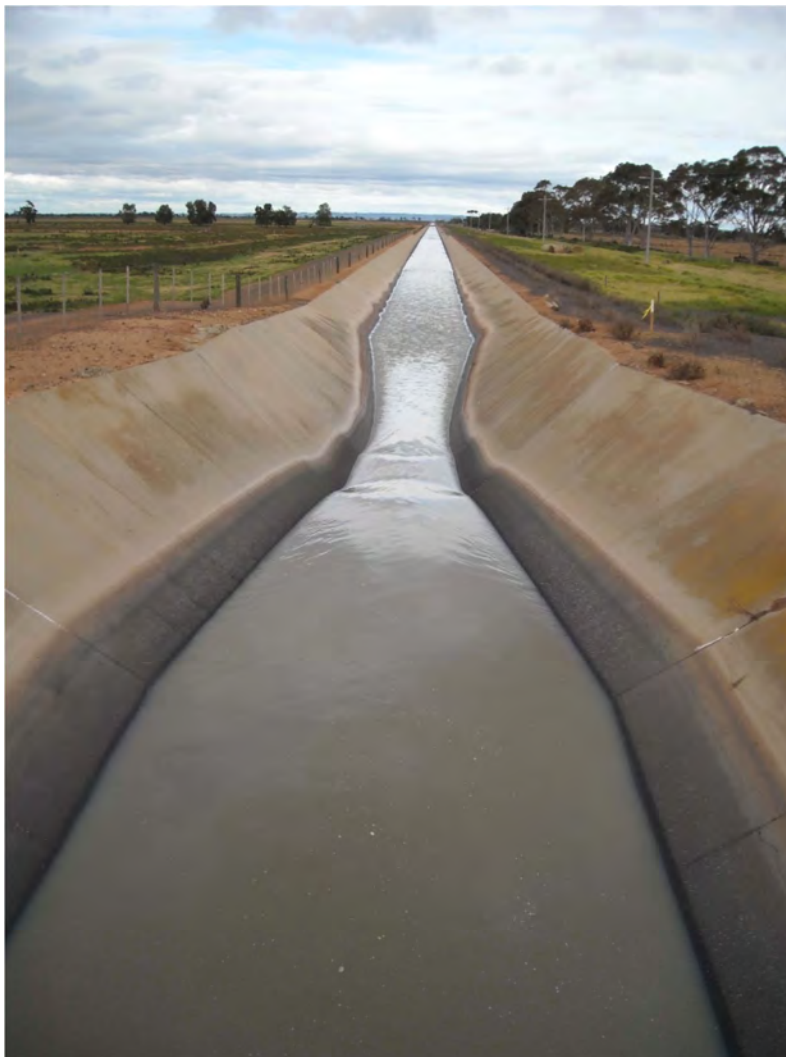
Figure 5: Photograph of existing long-throated flume
